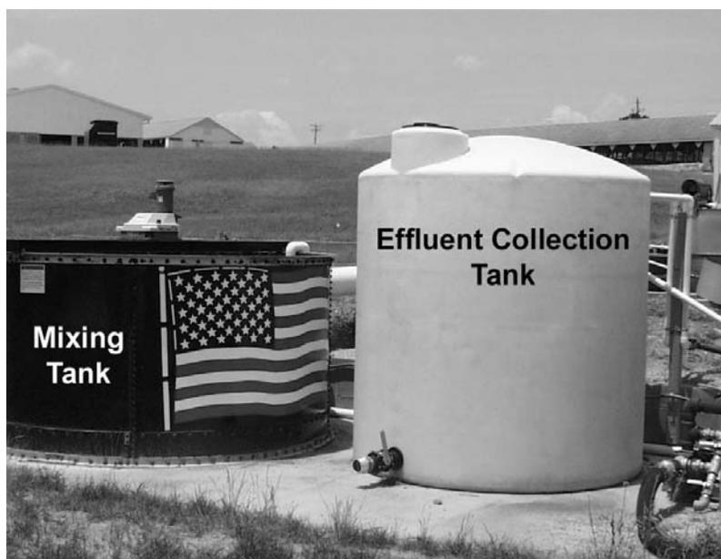
Figure 1. Influent and effluent tanks at the NCSU test site.
