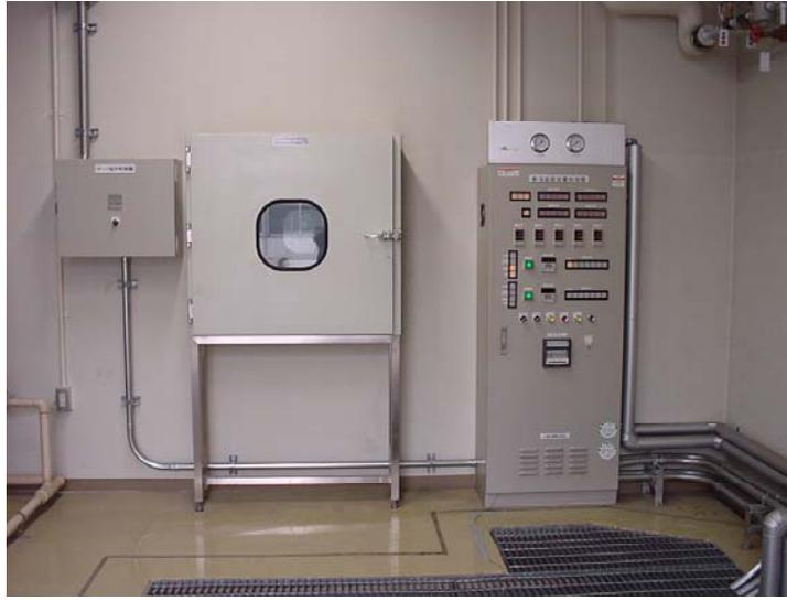
**Figure 7. Pass box and controller.**
