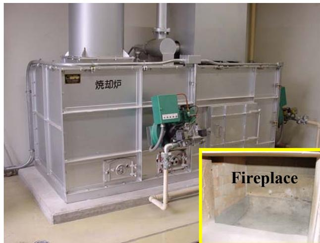
**Figure 6. View of incinerator and fireplace.**
